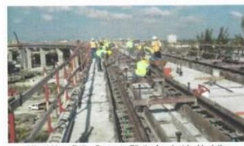
Miami MetroRail - Concrete Pilthns for electrical isolation
