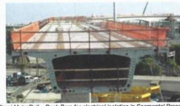
Miami MetroRail - Deck Bars for electrical isolation in Segmental Precast
